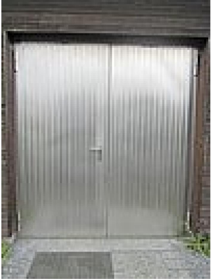
The door leaves and frame closing flush, the fixable and swing leaf opening to the outside (in escape direction).
