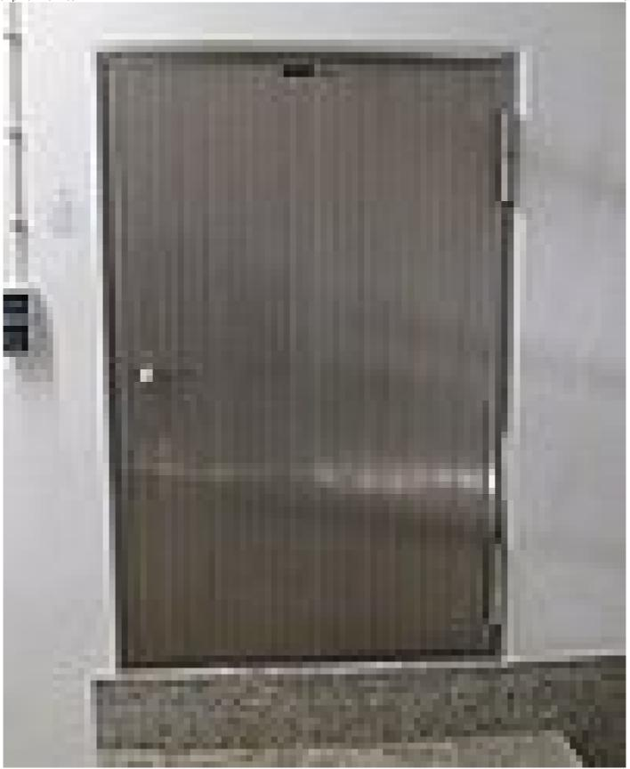
The door and frame closing flush, the door opening to the outside (in escape direction).
