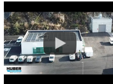
Video: Complete wastewater treatment at the Øygdalen WWTP in Norway https://www.youtube.com/watch?v=KU2awn3DP68
