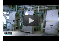
Video: RakeMax® Multi-Rake Bar Screen for mechanical preliminary wastewater treatment at a municipal WWTP
