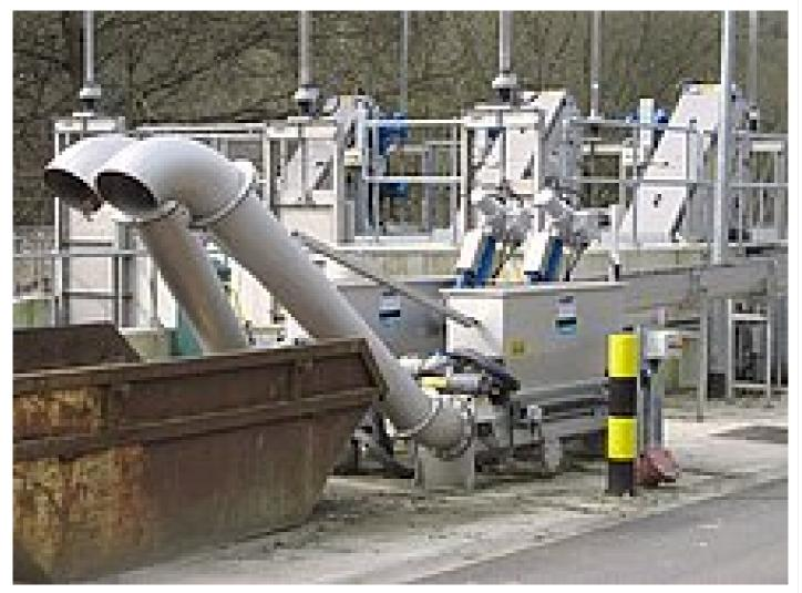
Screenings wash press for increased dewatering with launder channel feeding system
