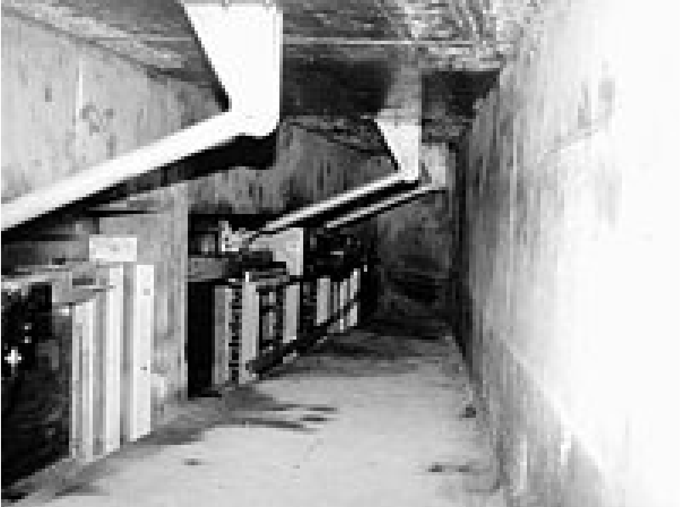
Facing adverse working conditions in the narrow building
