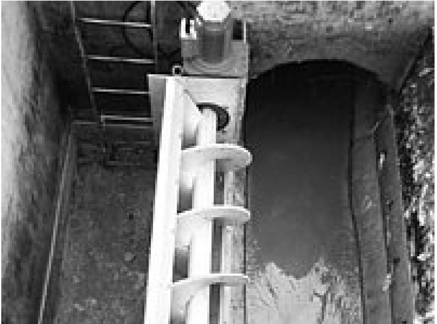
Screening of up to 10 m 3 /s combined water with 6 mm perforated plate
