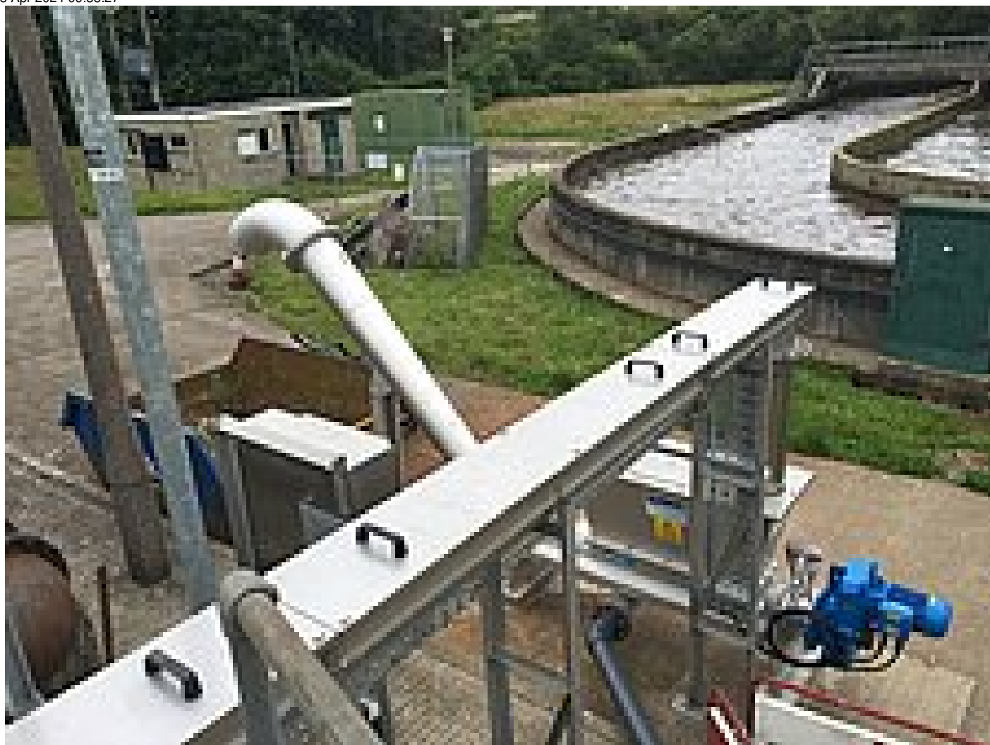
Launder Channel feeding the Wash Press
