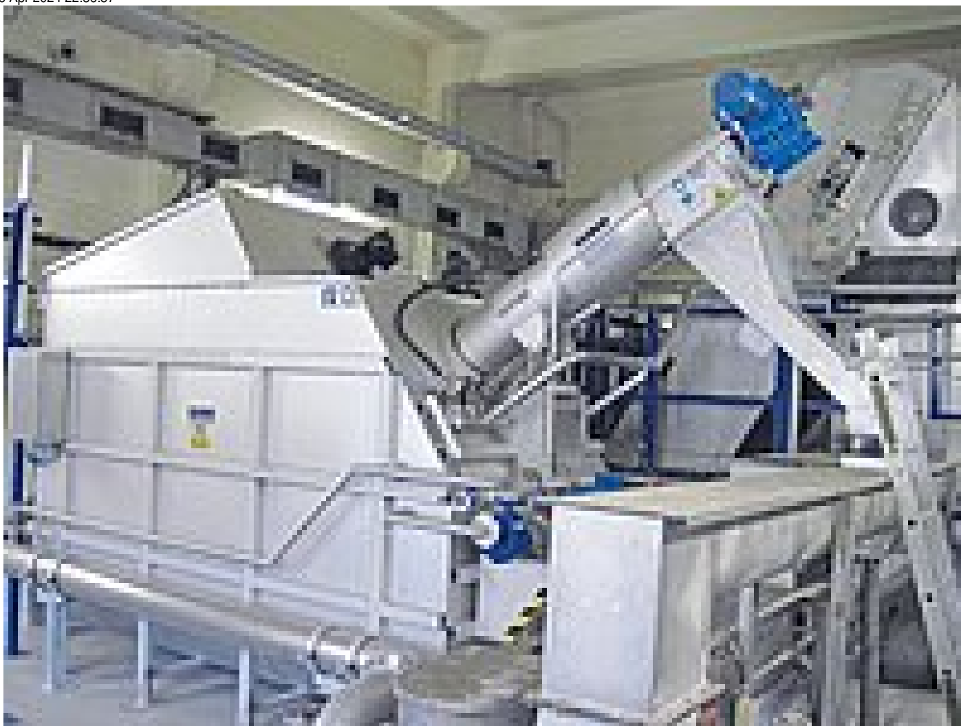
Discharge from the HUBER ROTAMAT® Membrane Screen RoMem
