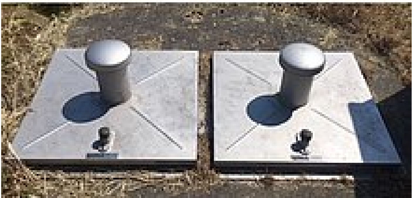
Figure 4. A galvanised cover vs HUBER stainless steel covers
