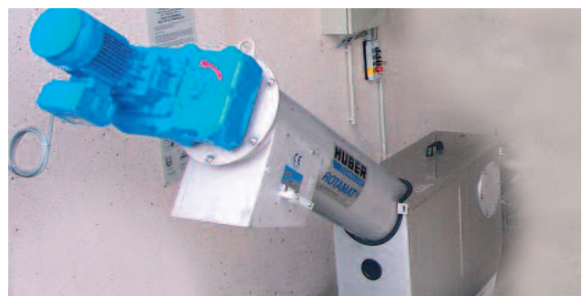
Tank-mounted ROTAMAT® Ro 9 Ec Screw Screen
