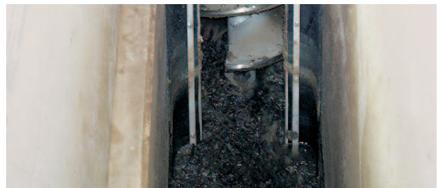
ROTAMAT® Ro 9 XL Screw Screen with maintenance-free ceramic bearing at the bottom
