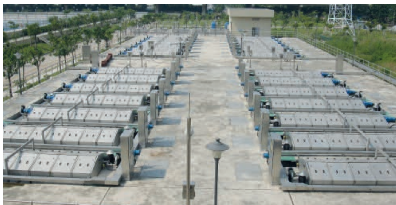
28 RoDisc® Rotary Mesh Screen units with 24 discs each treating about 8.5 m 3 wastewater per second
