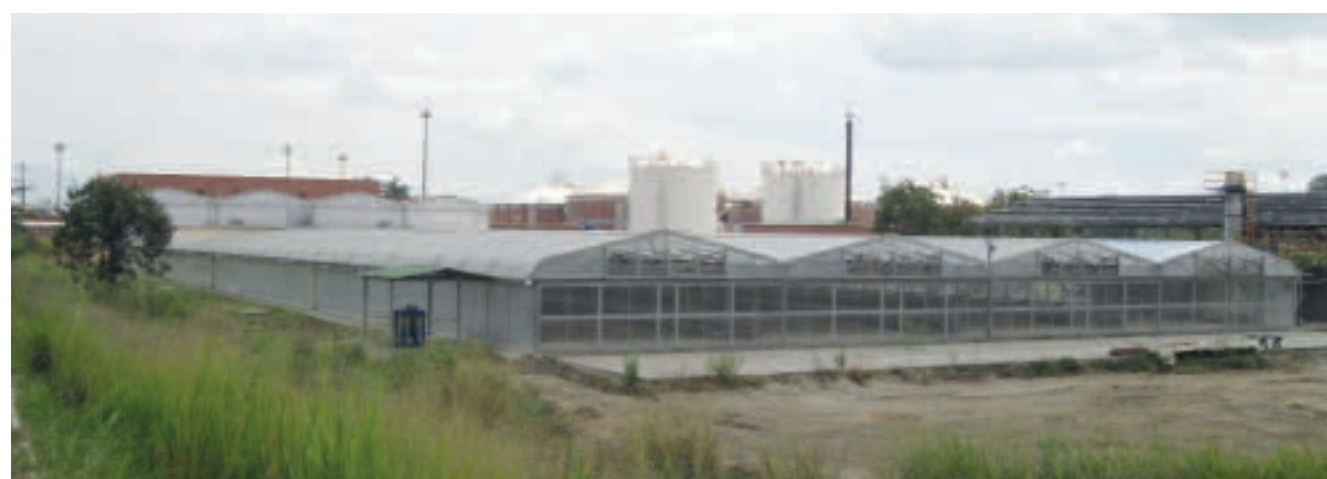
The sun makes sludge a valuable resource: the solar dryer at Cali produces fertilizer
