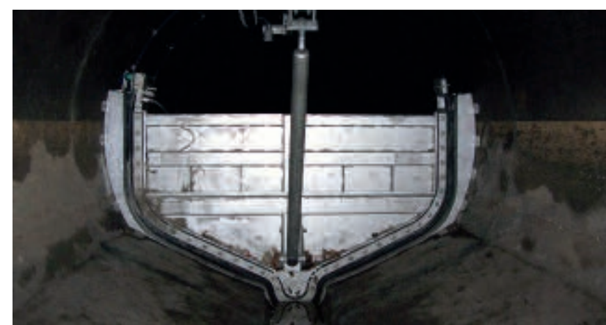
Flushing gate optimally adjustable to any sewer shape
