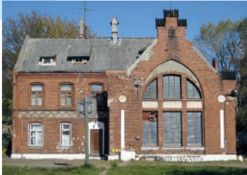
Wastewater pumping station, previous installation
