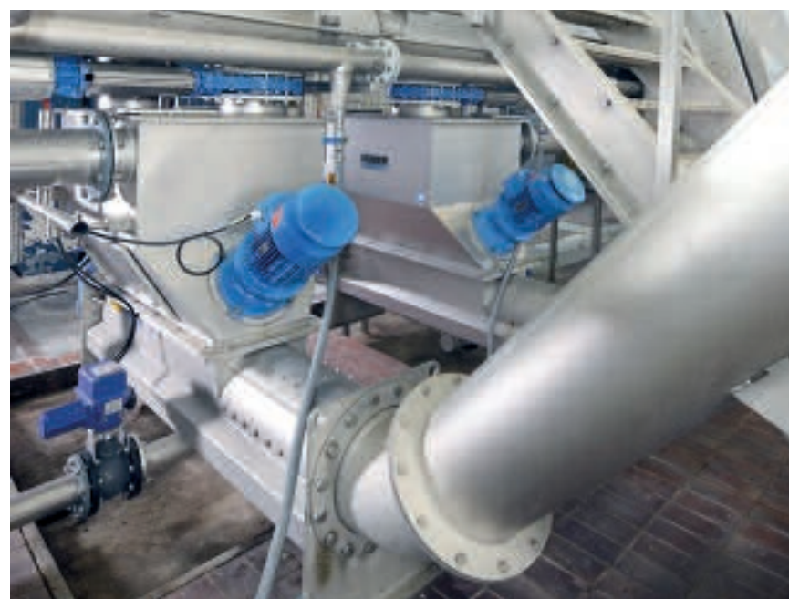
HUBER Screenings Wash Press WAP/SL units with powerful high-turbulence washing for throughputs up to 12 m 3 /h installed in Finland
