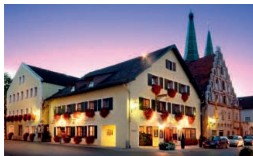
Four-star hotel Fuchsbräu in Beilngries, Germany (Fuchsbräu 2011)
