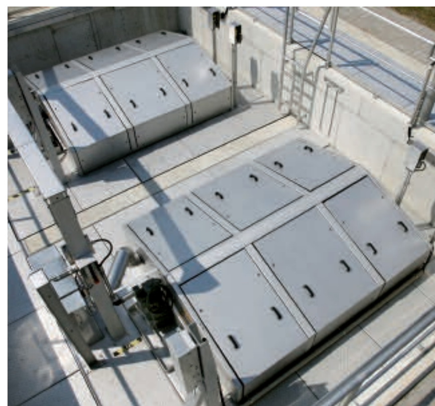
RoDisc® Rotary Mesh Screen for the retention of activated sludge flocks
