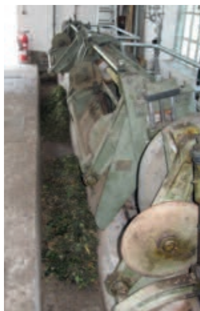
Fine screen system before replacement work
