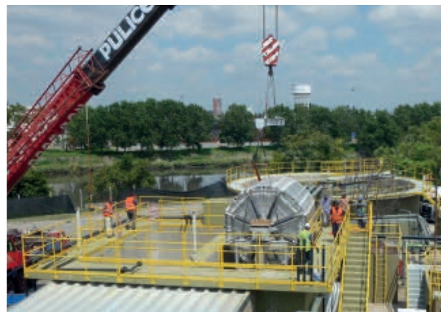
The two VRM® 30 / 480 units during installation into the membrane chambers
