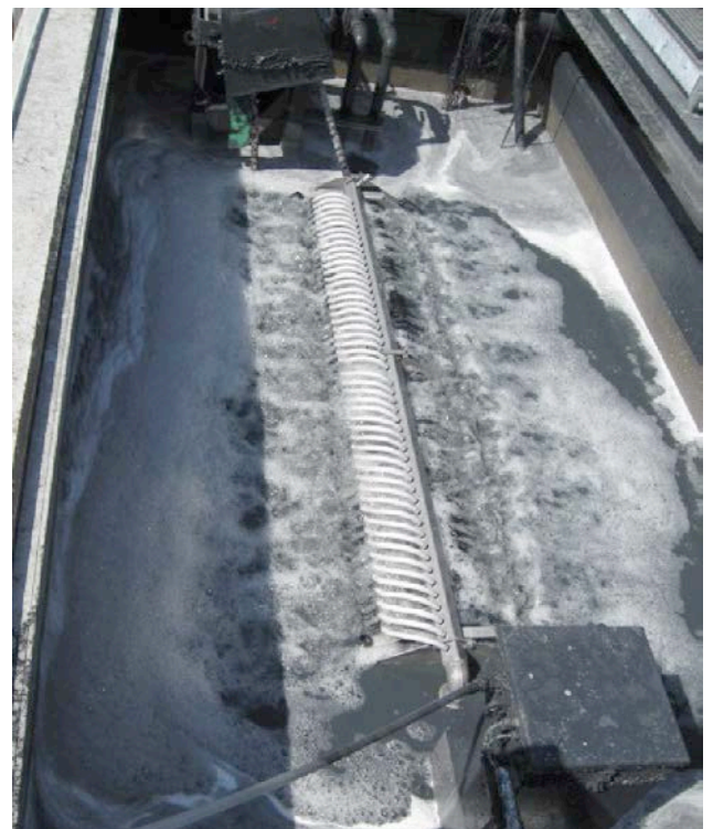
Scouring air introduction into VRM® plant
