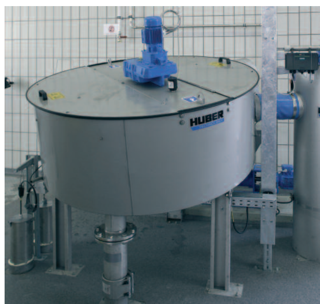
ROTAMAT® Disc Thickener RoS 2S
