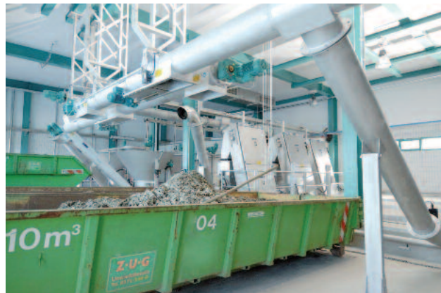
HUBER ROTAMAT® Screw Conveyor Ro 8t discharging screenings
