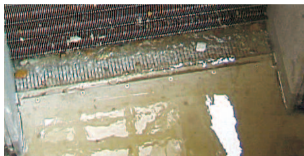
STEP SCREEN® with optimal bottom step design. The channel floor is flush with the top of the lowest step.
