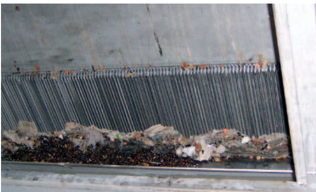
Bar rack with a spacing of 1/4 inch (6 mm); the bars have a streamlined tear drop profile resulting in low head loss and avoiding jamming; RakeMax screens are unimpaired by grit and gravel
