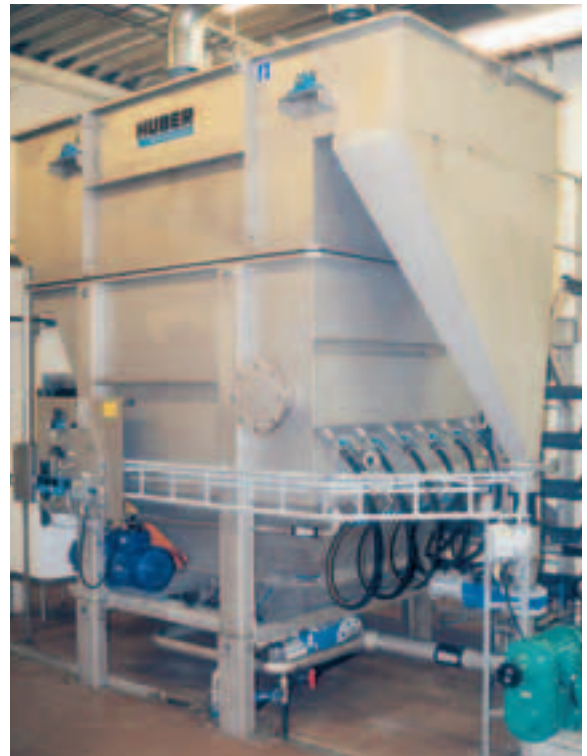
SWE-DAN Seafodd / fish industry, Västervik/Sweden, HUBER Dissolved Air Flotation Plant HDF-3 with chemical treatment, throughput: 66 GPM (15 m 3 /h)
