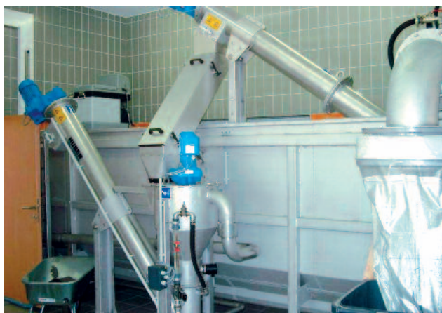
Classifying screw with subsequent HUBER Coanda Grit Washer RoSF4 T
