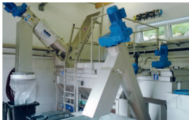
Complete Plant with integrated Grit Washer
