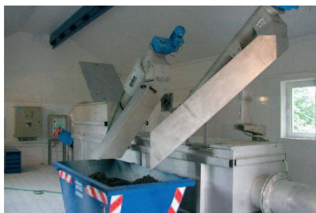
ROTAMAT® Complete Plant Ro 5K with integrated cross-flow lamella separator
