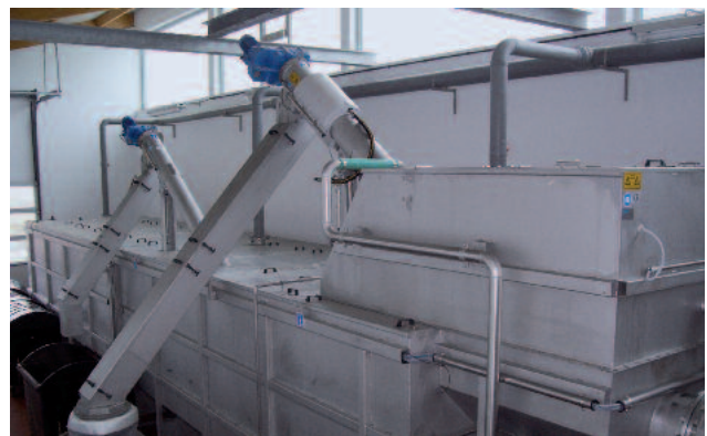
Odour-free, clean screenings and collected grit discharge
