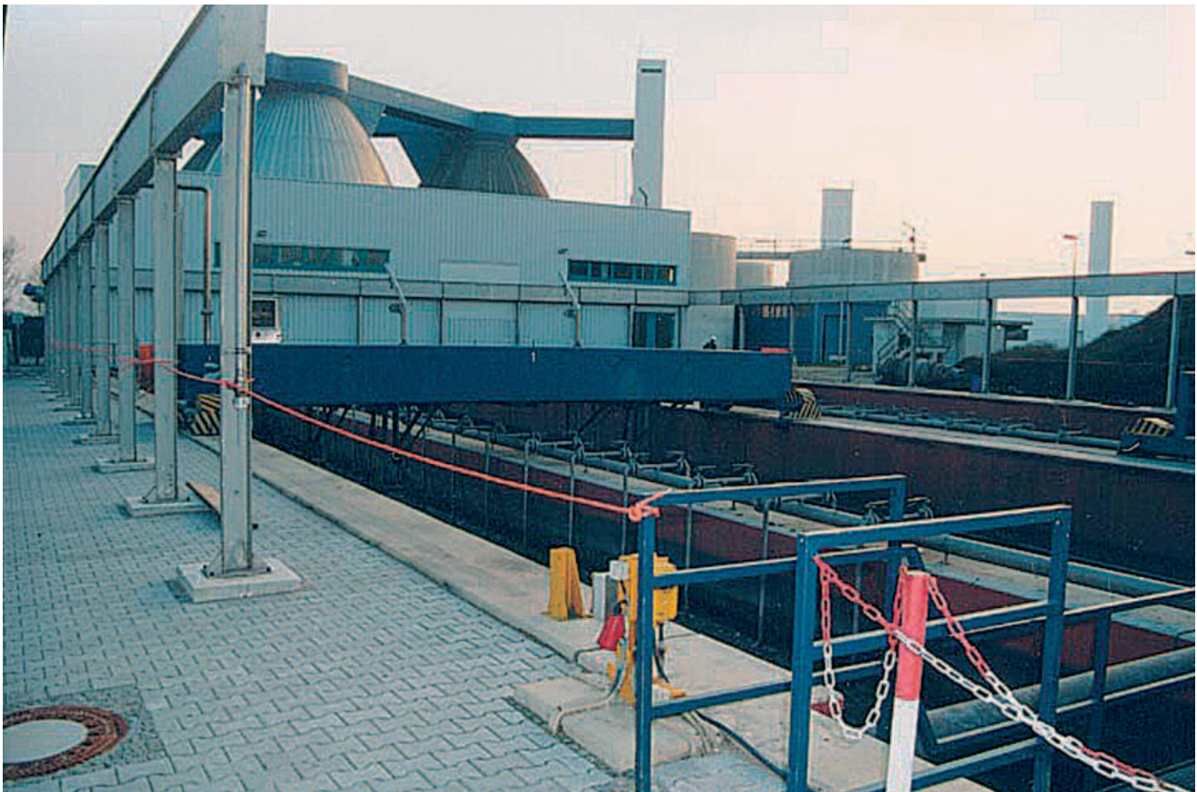
Typical longitudinal grit trap with suction clearer
