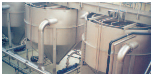
HUBER HRSF Grit Traps installation
