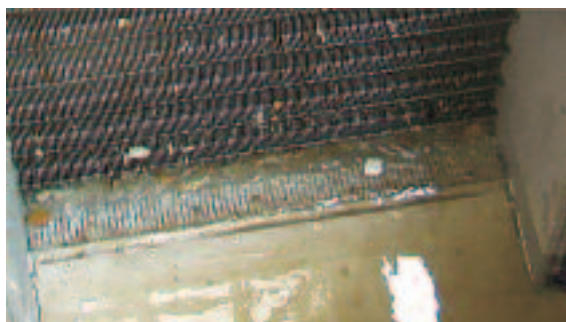
STEP SCREEN® with optimal bottom step design. The channel floor is flush with the top of the lowest step.
