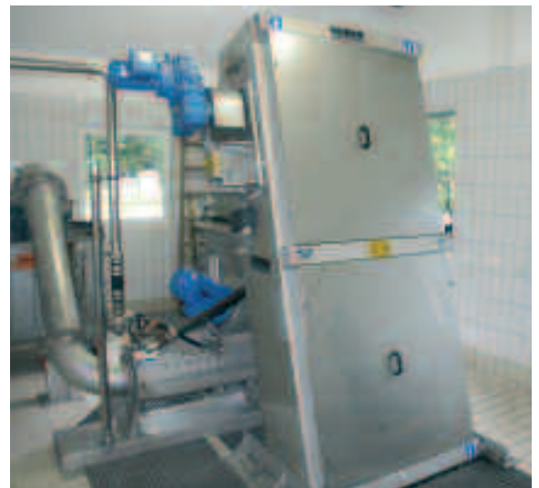
1/4 inch (6 mm) RakeMax feeding into a Super-Launder Washpress WAP/SL for perfect screenings washing and compaction
