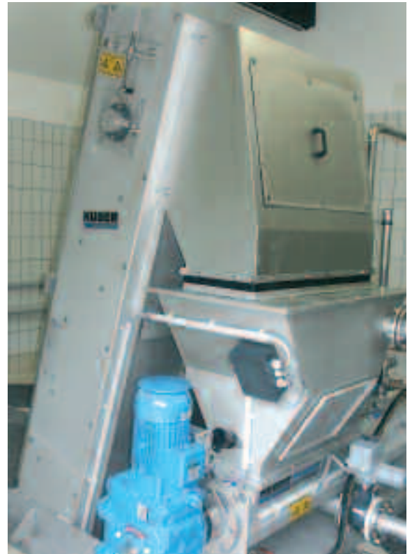
Complete enclosure for odor protection; the chain tensioning system is visible at the side of the frame
