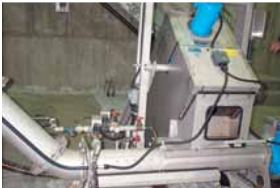
Wash & Press WAP Washing, compaction/dewatering and conveying of screenings with volume and weight reductions of up to 70%.
