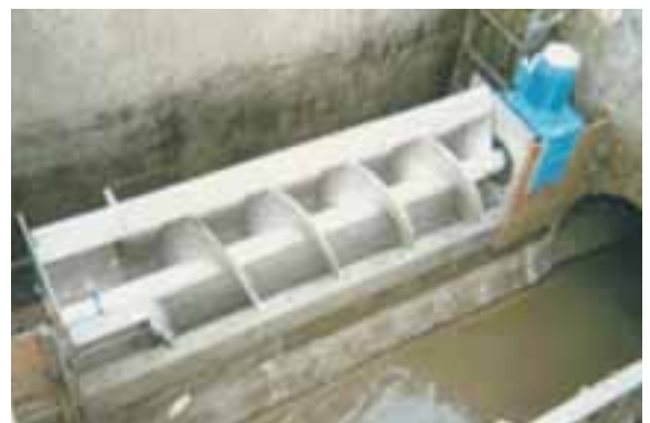
ROTAMAT® Stormwater Screen RoK 1 Removes solids larger than 1/4" in CSO's. Units are available to handle flows from 1 MGD - 240 MGD!
