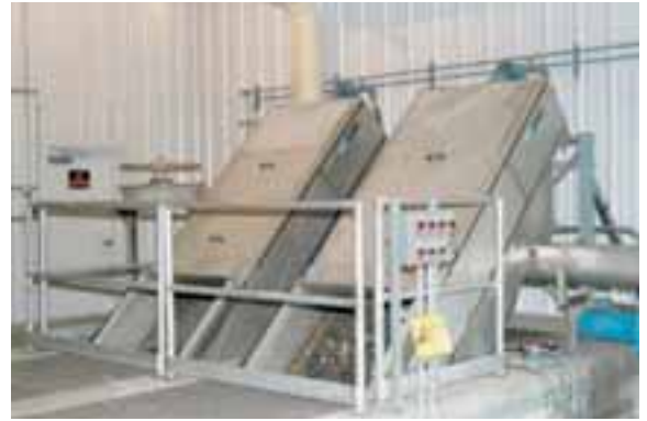
STEP SCREEN® The STEP SCREEN® is a well-proven fine screen for water, wastewater and industrial effluent. Variable installation angles permit installation into almost any channel.
