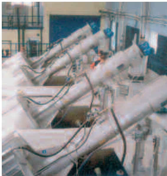
Four ROTAMAT® Rotary Drum Fine Screens provided with integrated screenings washing (IRGA)
